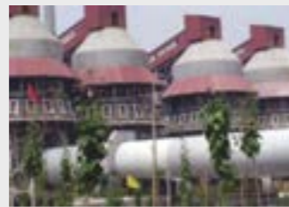
Anshan Iron and Steel Group Corporation 1000TD Rotary Kiln in Bayuquan
