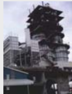
The 600t Maerz PFR Kiln of Mayes Steel Plant in Malaysia
